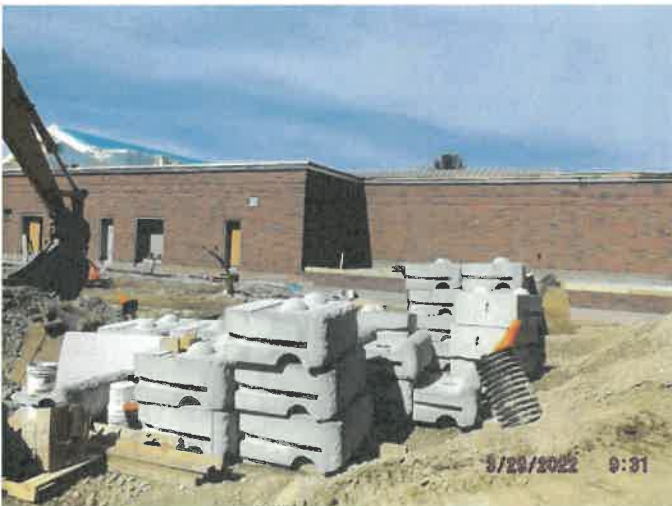
Photo depicts the progress of brick installation at rear of site.
