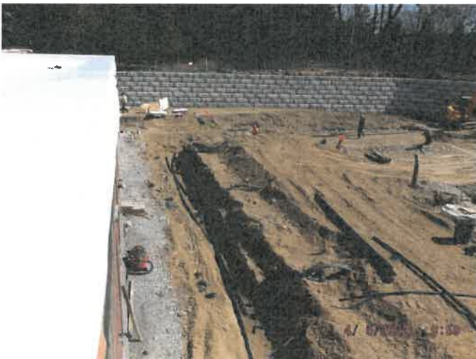
Photo depicts the progress of the retaining wall and geo-thermal
