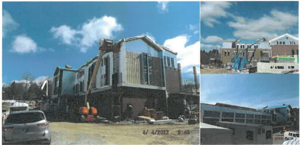
Pictures: Overall Site Progress
