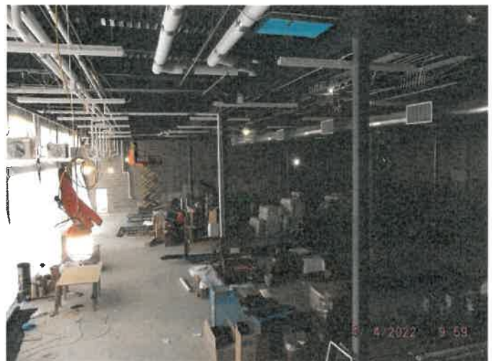
Photo depicts the progress of the apparatus bay.
