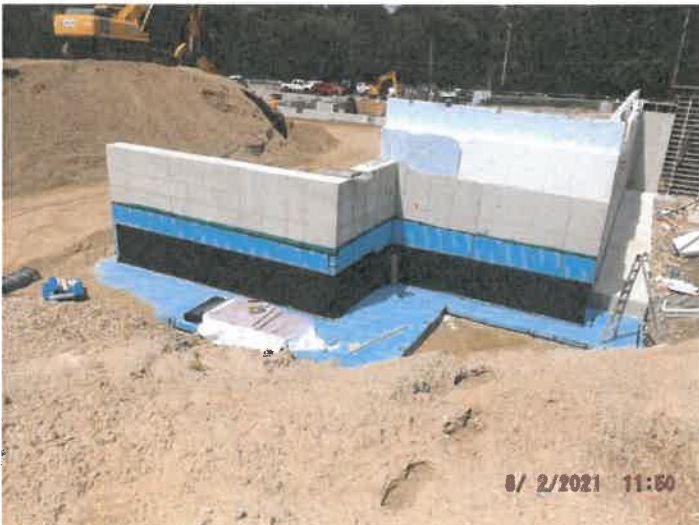
Photo depicts the progress of waterproofing.
