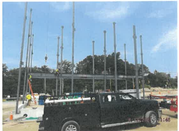
Photo depicts the steel erection.
