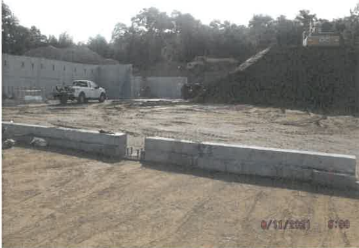
Photo depicts the site progress along with footing and foundation progress.
