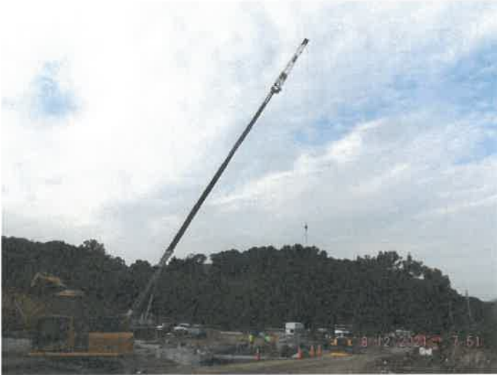
Photo depicts the arrival of the crane for steel.
