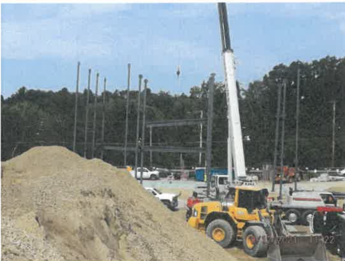
Photo depicts the steel erection.
