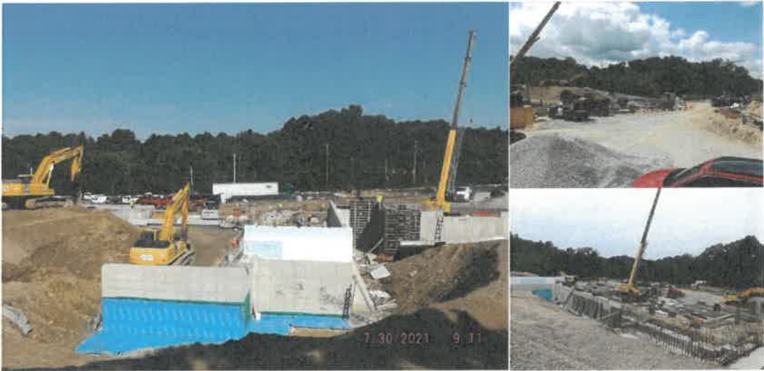
Pictures: Overall Site Progress
