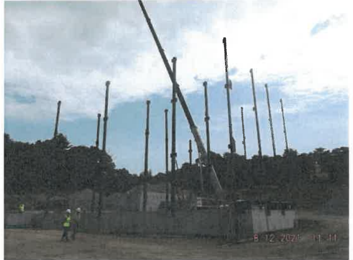
Photo depicts the steel erection.
