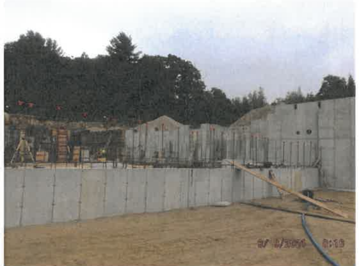
Photo depicts the progress of high wall panel installation.
