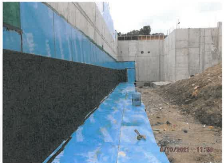
Photo depicts the progress of waterproofing.
