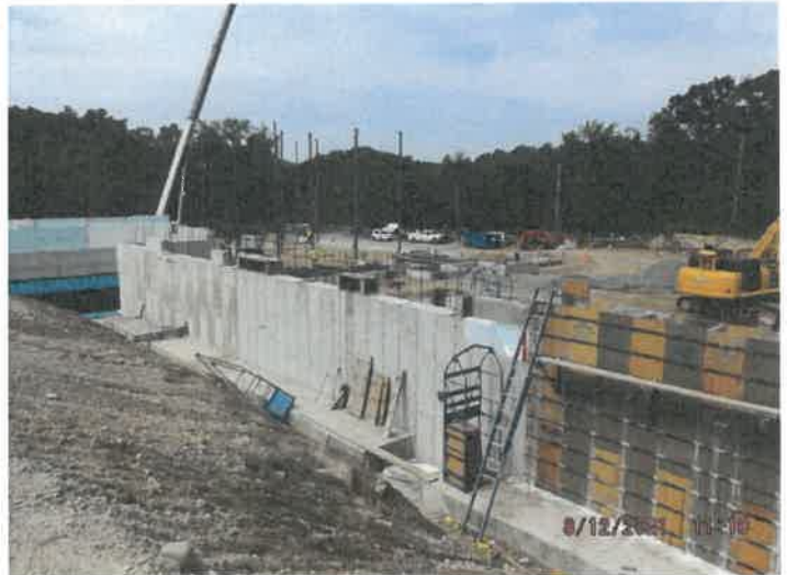
Photo depicts the site progress along with footing and foundation progress.
