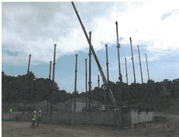
Photo depicts the steel erection.
