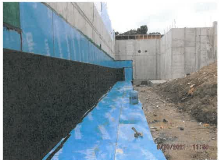
Photo depicts the progress of waterproofing.
