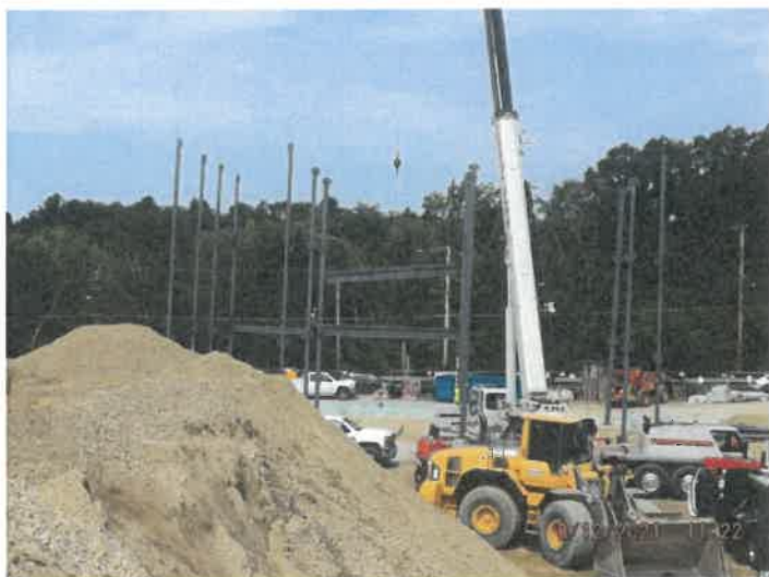
Photo depicts the steel erection.
