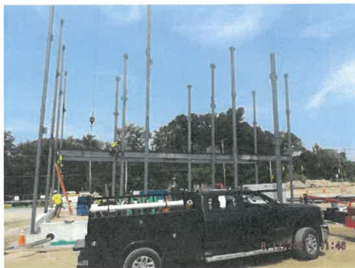
Photo depicts the steel erection.
