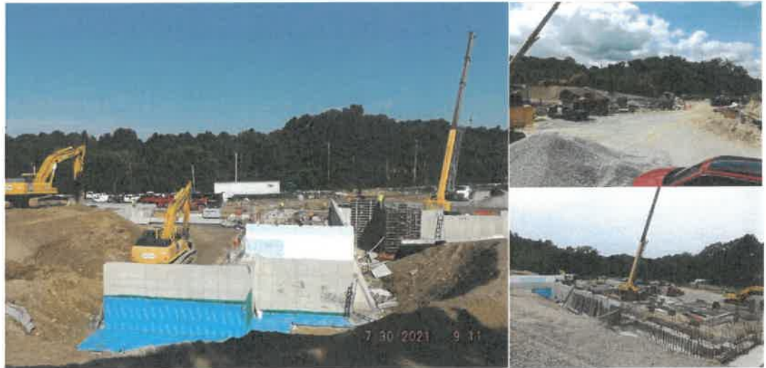
Pictures: Overall Site Progress
