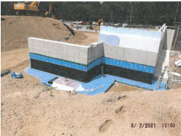
Photo depicts the progress of waterproofing.
