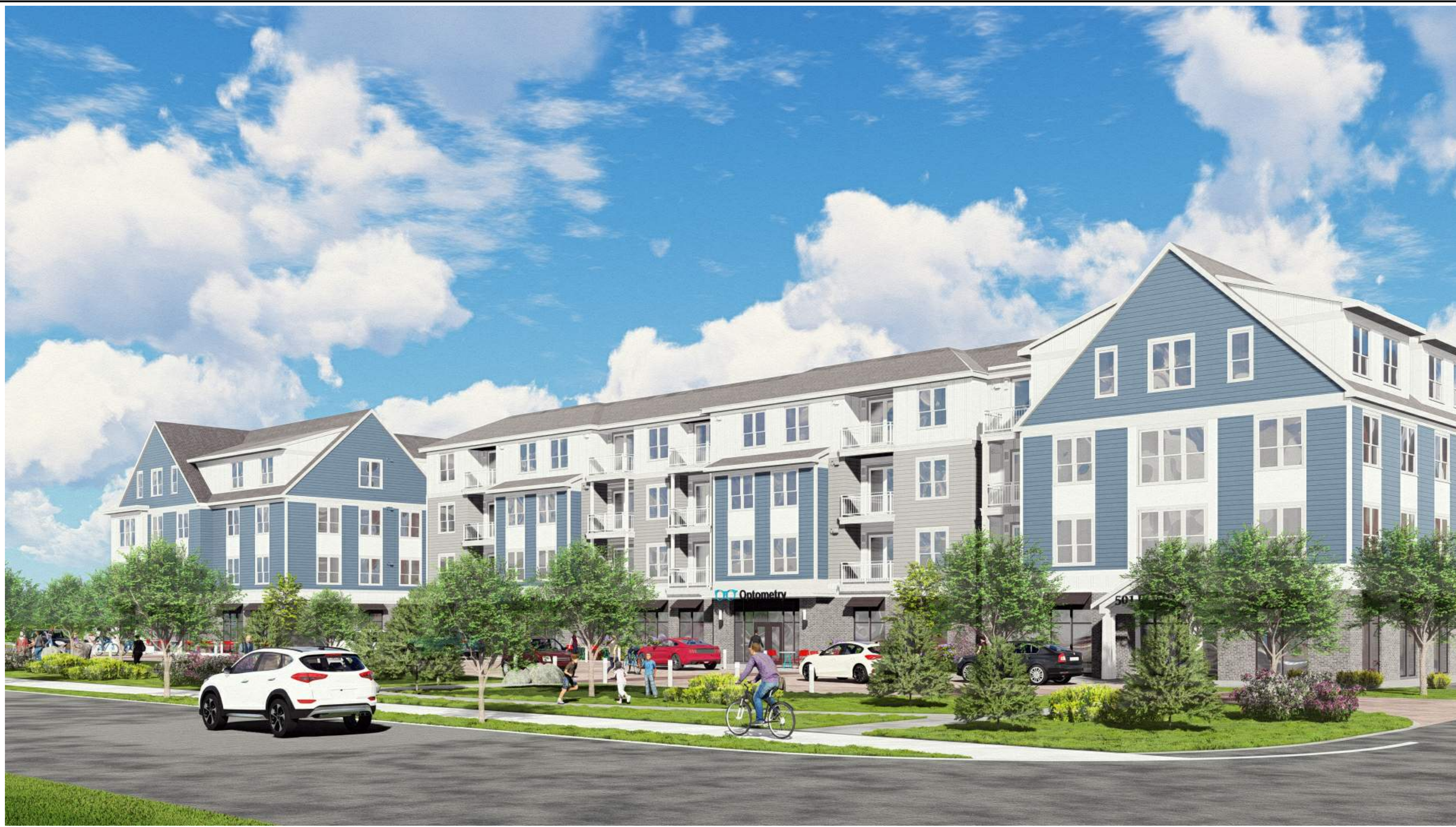
VIEW FROM POND STREET - BUILDING ENTRY
