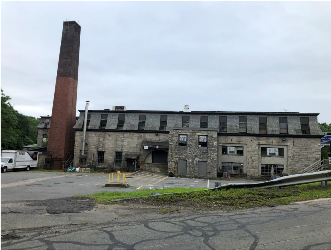
10-20 Main- Top photo – small 2 story appendage at center to be removed
