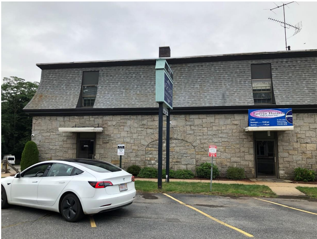
10-20 Main Street – circa 1870 – to be renovated in place
