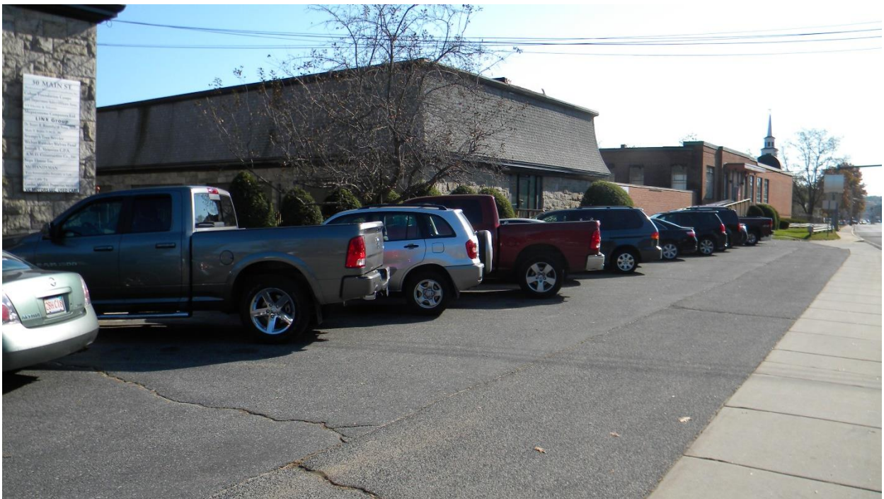
40 Main Street – general front view
