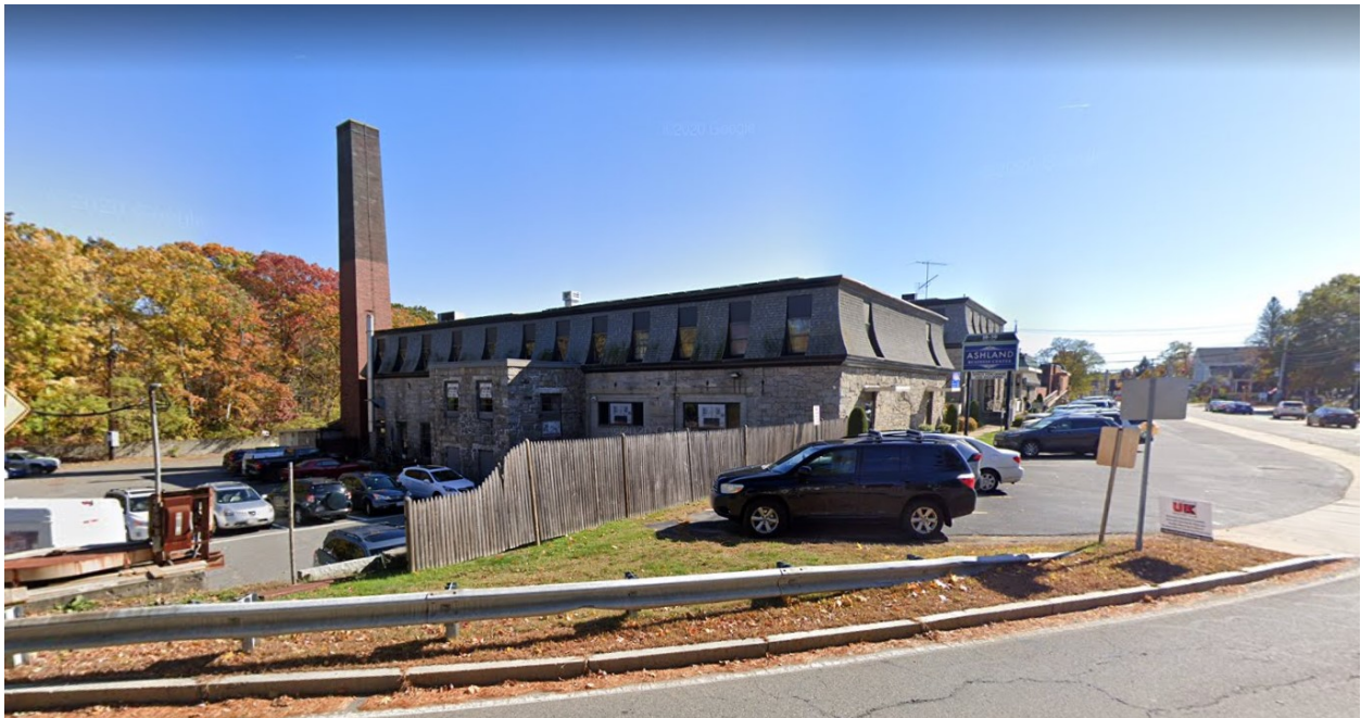
Current view of 10-50 Main from Myrtle Street. Source: Google Maps.
