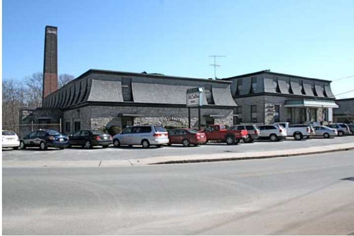
View SE: 10 Main (left, ASL.200) and 30 Main (right, ASL.201)
