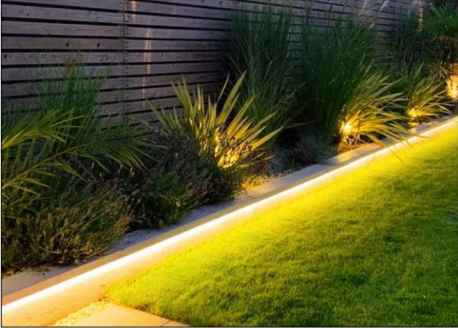
IN-GROUND LED STRIP LIGHTING
