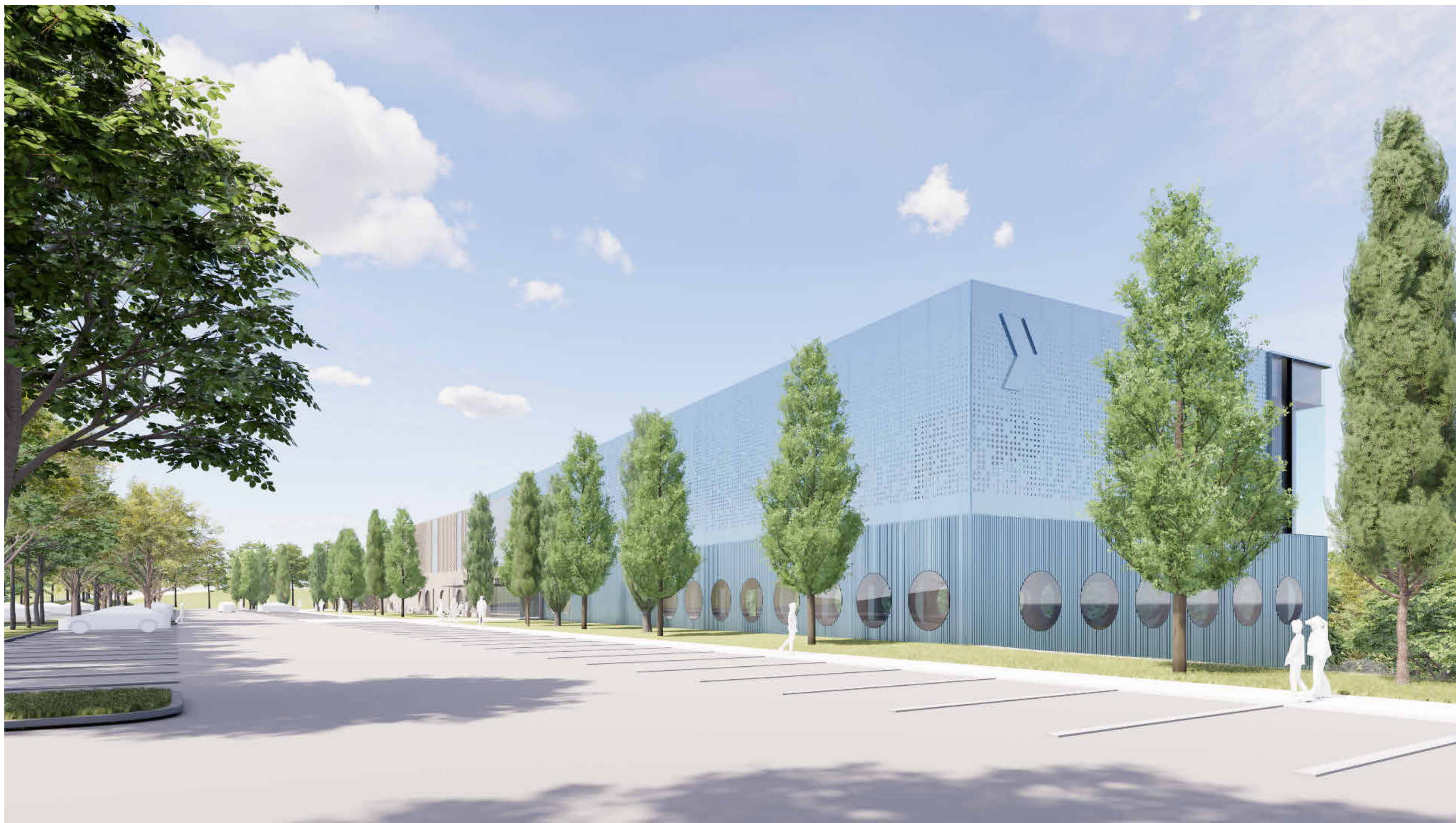
VIEW FROM ENTRANCE OFF MEMORIAL DRIVE- SOUTH EAST CORNER
