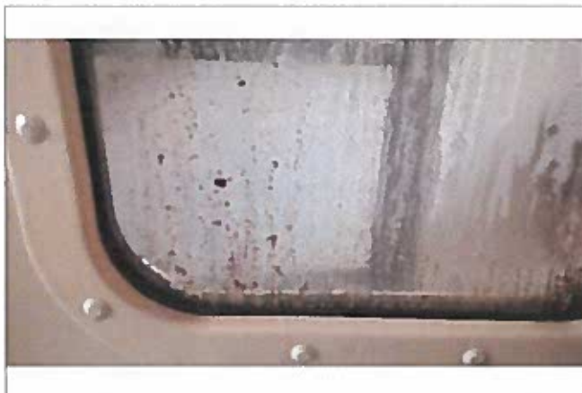
Produce door window with what appears to be mildew
