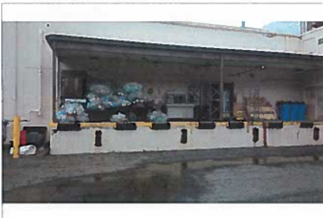
Rear loading dock. Remove all refuse.
