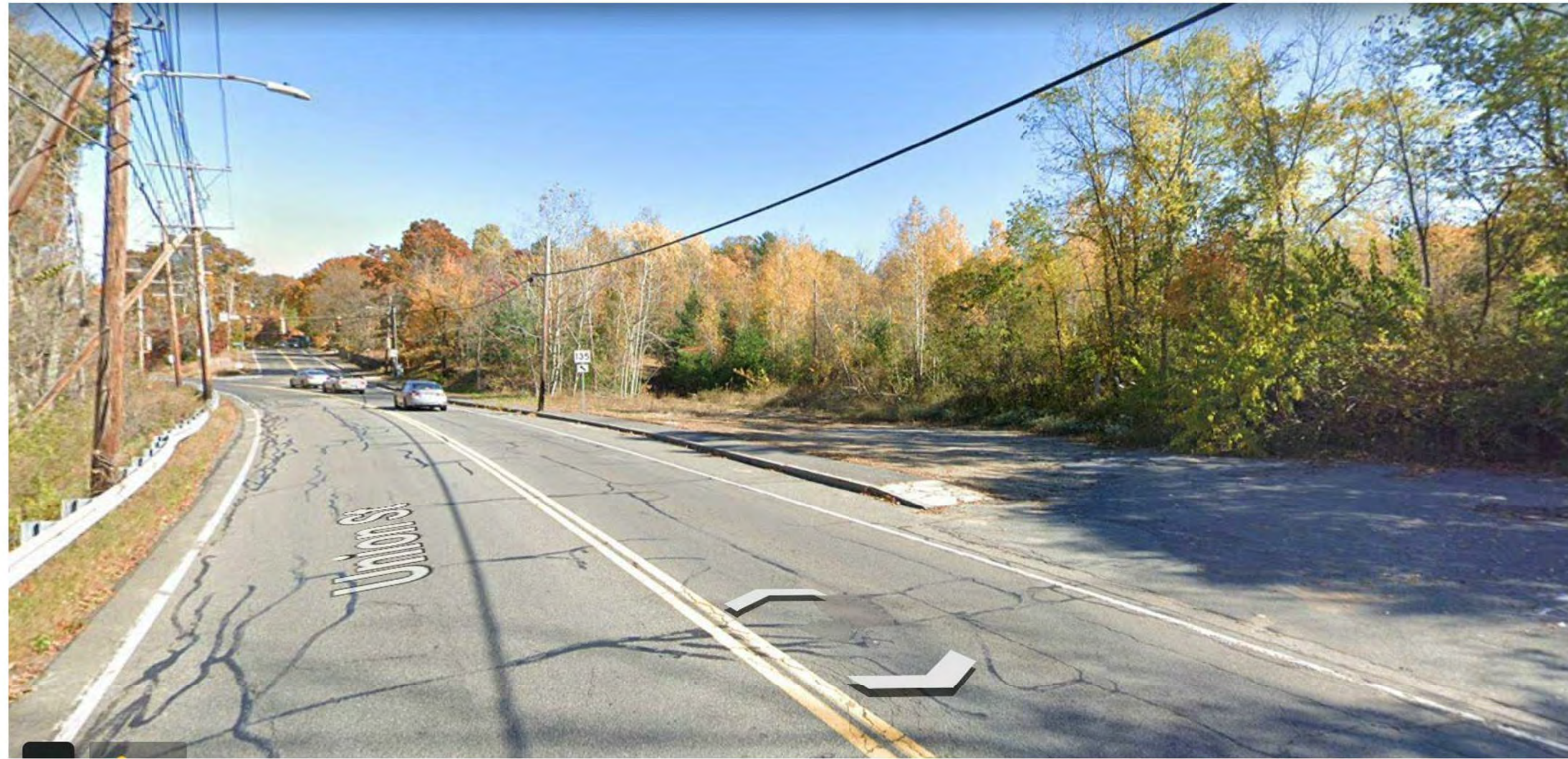
A - VIEW LOOKING EAST ALONG UNION STREET
