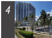
4 Campo Felice Fort Myers, FL 323 Apartments
