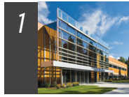
1 United STEP I Malta, NY Office Space, Light Manufacturing 105,000 Square Feet
