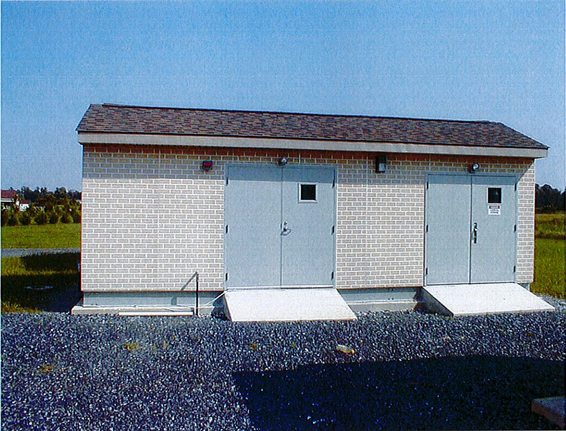
Typical Prefabricated Booster Pump Station Buildings Manufactured at a factory, shipped to site and installed on concrete pad.
