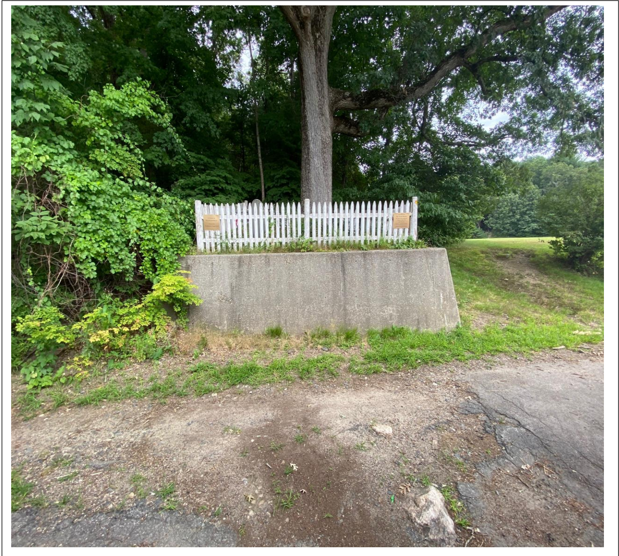
Cement retaining wall at +-10' from the center of tree
