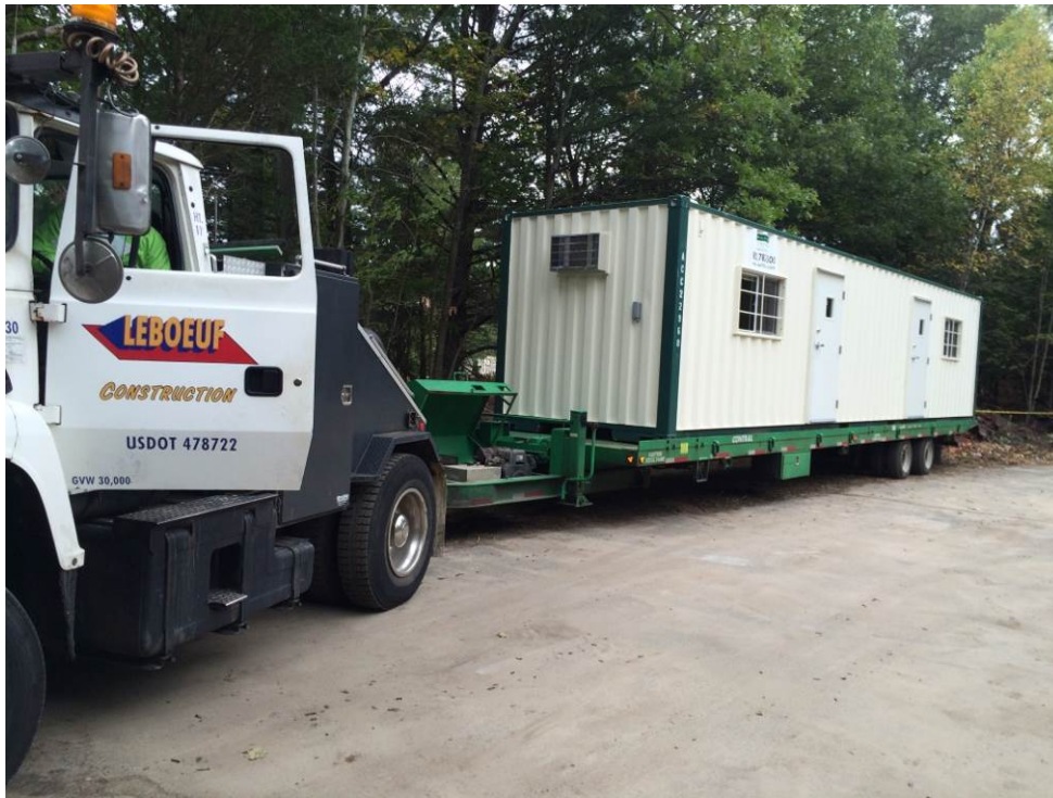
SCENE: View of the office trailer being delivered to site. Photograph taken facing southeast.
