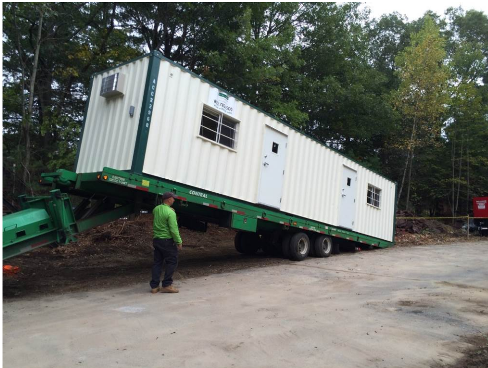
SCENE: View of office trailer being unloaded. Photograph taken facing southeast.
